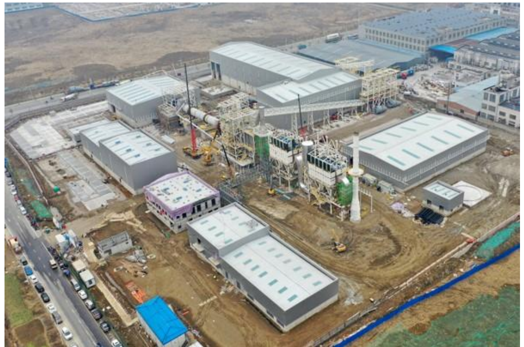
↑ Changzhou construction site, early February 2021
