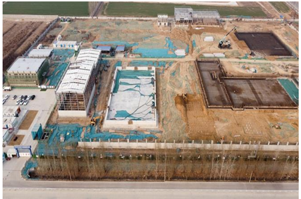
↑ Xuchang construction site, January 2021
