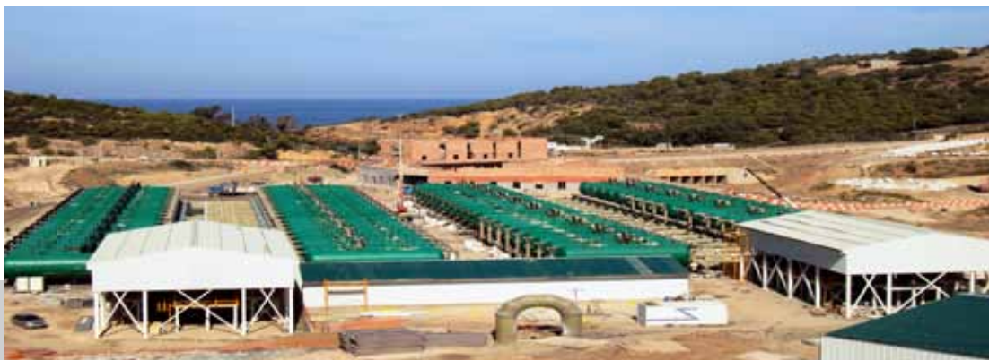
Outside view of the Desalination plant in Honaine (Algeria)
