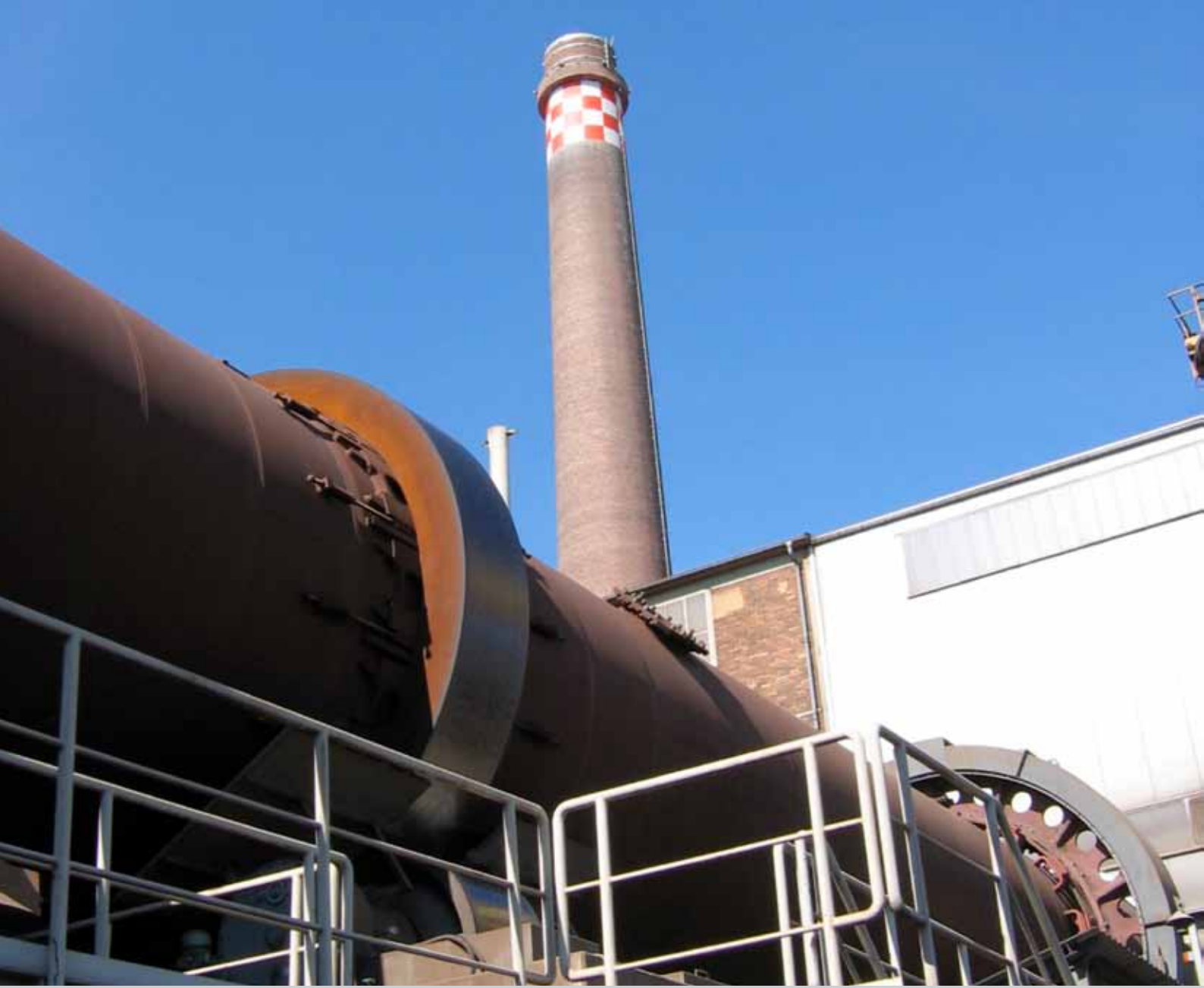
Lateral view of the Waelz furnace from Befesa Zinc Freiberg (Germany)
